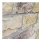
The most common grout technique is a **standard or raked joint**. This is what you typically see with brickwork, for example. The grout is evenly applied around the edge of each stone or brick. When finished,
