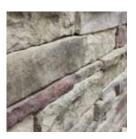
Many homeowners now choose the **dry stack** style of stonework, which is actually groutless. Mortar is used behind the stone to secure it in place, but there is no grout visible between the stones. This gives the work a very natural, casual appearance.
