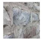
For a more old-world look, choose **overgrouting**. This technique uses a much heavier grout seam. Depending on the look you want, the grout can be even with or extend beyond the face of the stone, rather than being recessed like the standard
