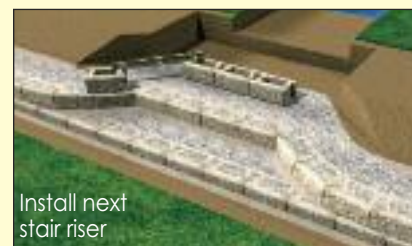
Backfill and compact
